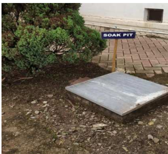
Figure 4: Soak pit for chemistry lab discharge
